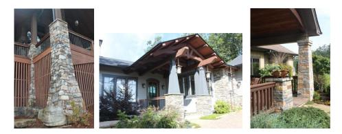
Columns on porches shall be round, square, or square-tapered; corners may be chamfered. Porches that are larger in proportion to the house must present a substantial look to the box columns.
